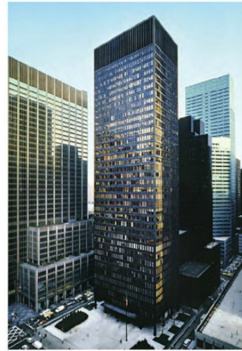
Fig. 15-42 Ludwig Mies van der Rohe and Philip Johnson, Seagram Building, New York City, 1958. © Andrew Gam.
